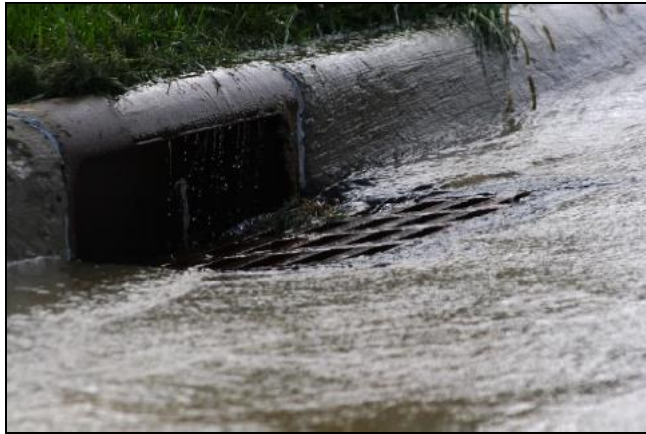
Storm water management
