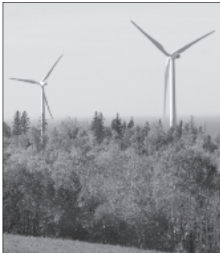
Wind turbines. Photo credit: Chantal Laliberté
