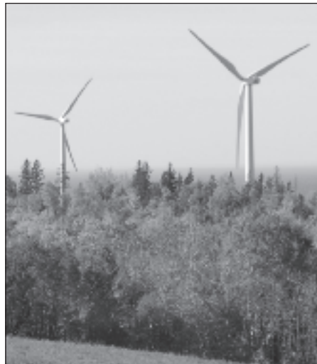
Wind turbines. Photo credit: Chantal Laliberté
