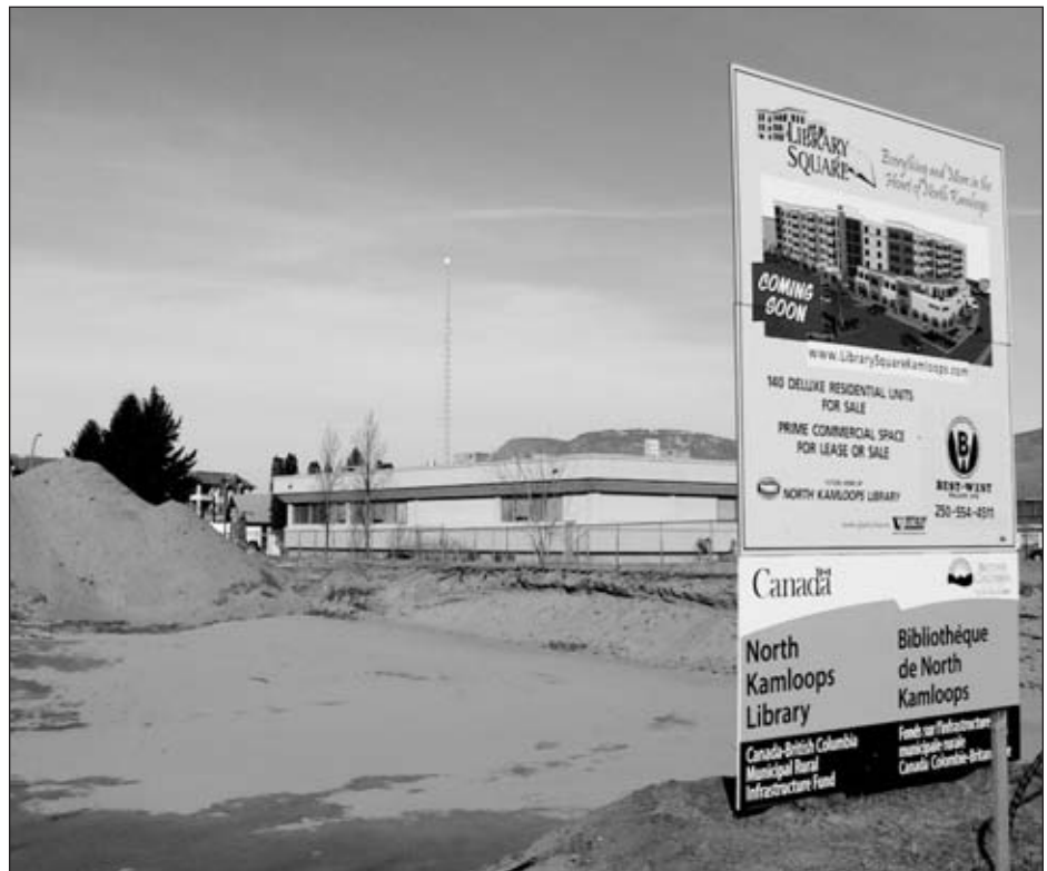
View of mixed-use development site within the North Shore's Towne Centre.
