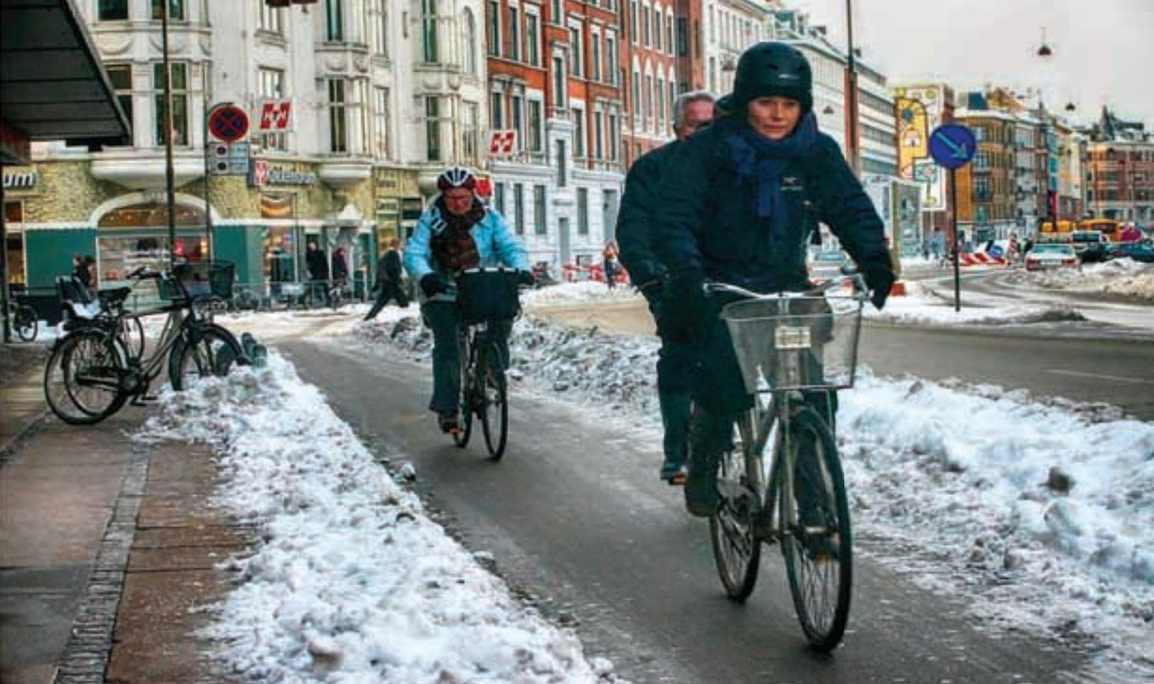
Above: Snow storage area included between roadway and elevated/raised cycle track and sidewalk, Copenhagen, Denmark. Source: Karhula K, 2014.
